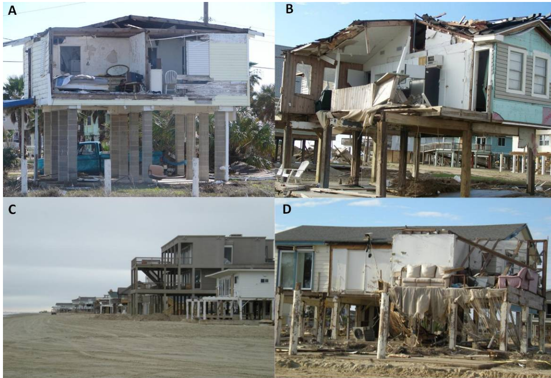
Figure 1. Damage caused by Hurricane Ike on Galveston Island. A. A house with its side ripped off. B. Destruction along the beach. C. A first row of houses was completely destroyed, leaving this second row as beachfront property. D. Remnants of a beach front house on the west end of Galveston Island.
