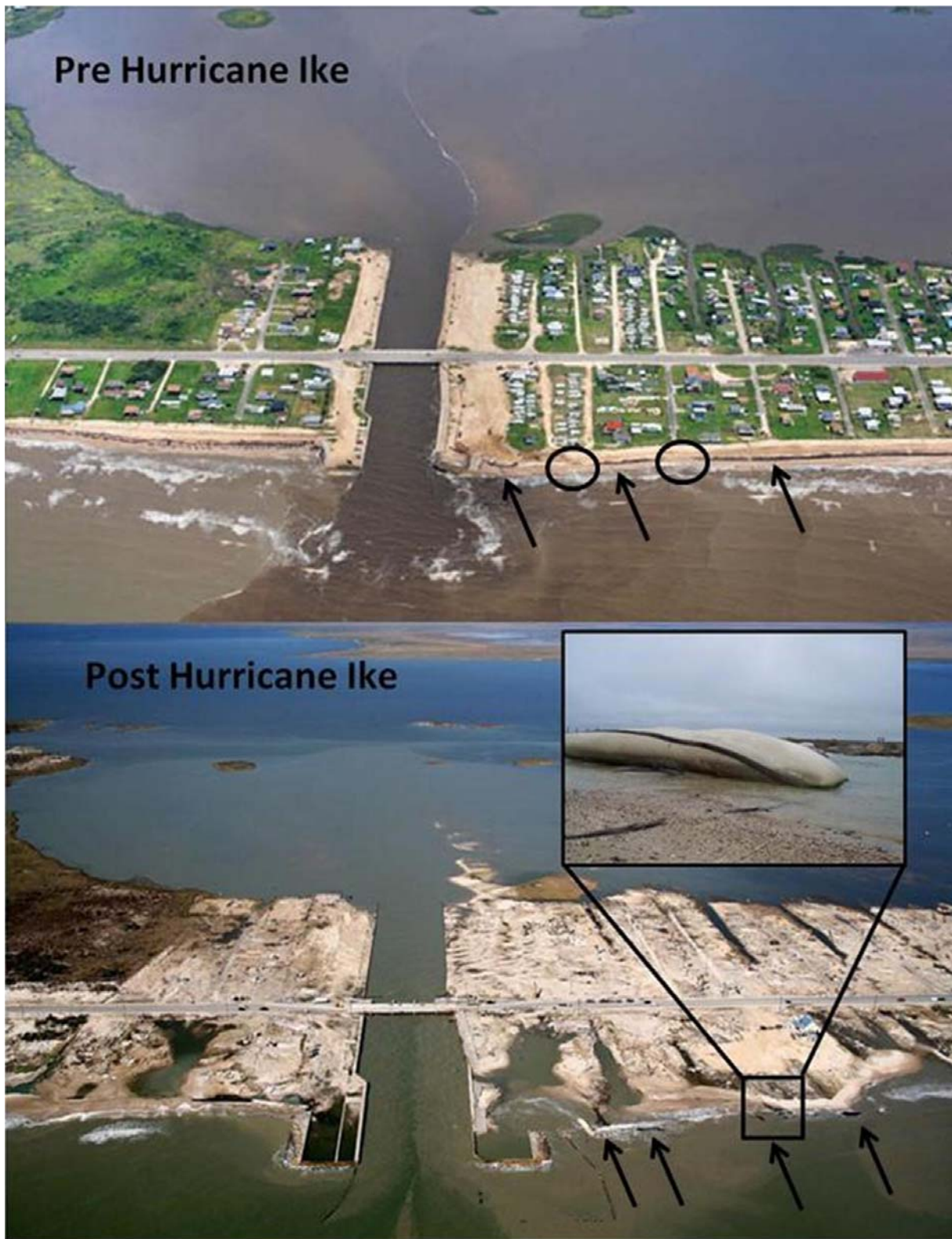
Figure 2. Aerial view of Bolivar Island pre- and post -Hurricane Ike (Texas General Land Office website). Arrows point to the locations of geotubes. Overwash fans in the post-hurricane image
