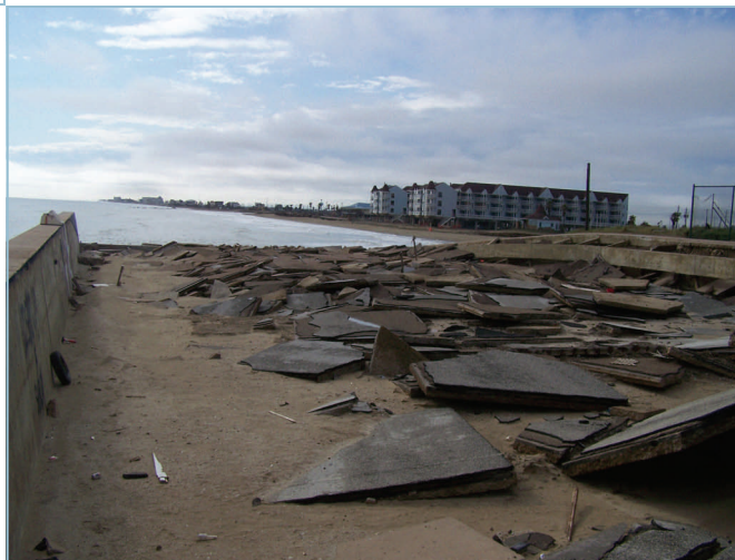
End of sea wall, Galveston Island, Texas.
