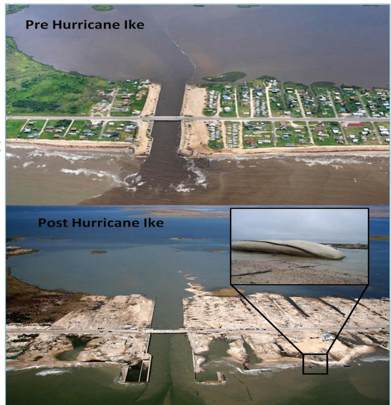
Figure 2. Aerial view of Bolivar Island pre and post Hurricane Ike (Texas General Land Office website). Overwash fans can be seen corresponding to the geotextile tubes. Inset is an on-the-ground picture of the destroyed geotextile tube (photograph by Heather Joesting).
