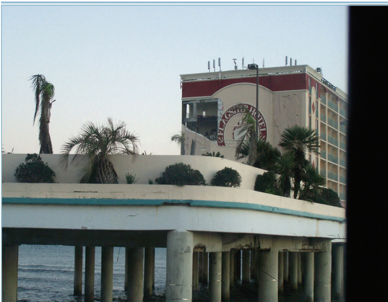
Hurricane Ike damage on the Flagship Hotel, Galveston Island, Texas.
