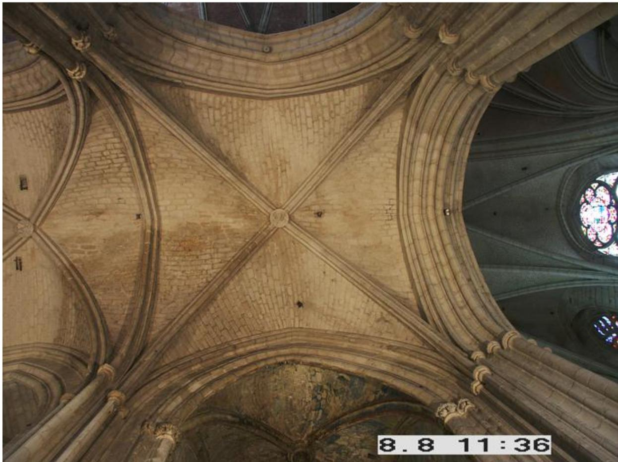
The *voutains* (as I will term the sections of the vaults, sometimes called in English severies, singular severy) are not uniform due the varied cross sections of its surrounding arches. The coursing of the voutains does not consist of standardized masonry blocks. As the masonry bocks approach the crown lines of the vaults, a series of *ad hoc* adjustments in individual blocks were made to close the vault. The vaults do not follow the curvature of the bounding arches in most cases.
